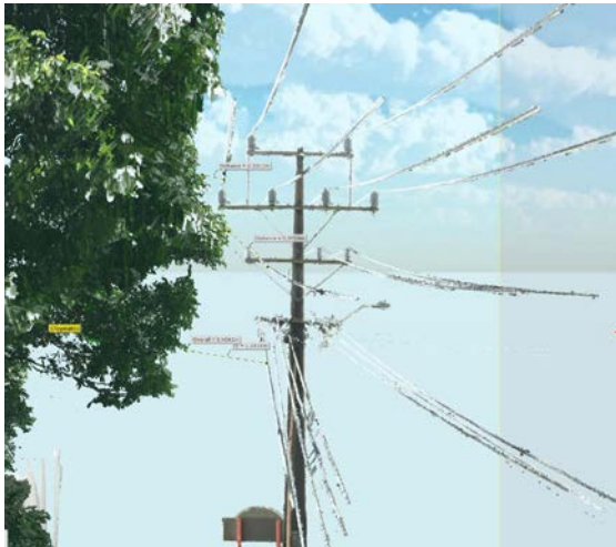
Vegetation clearance safety inspections
