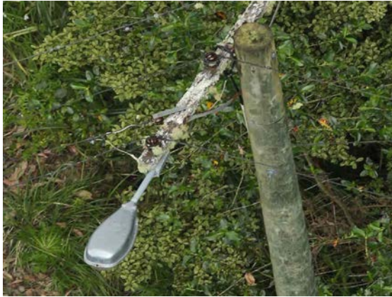
Pole top inspections
